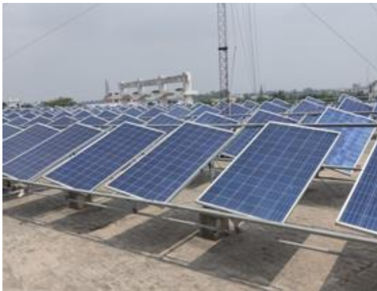
Solar Panel Installation
